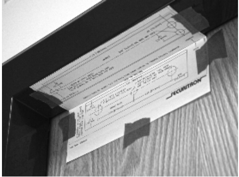
Figure 4. Attaching the Template
