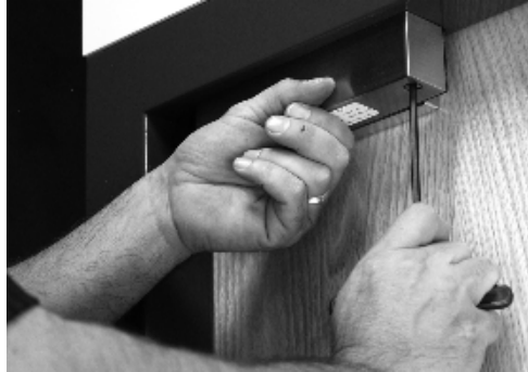
Figure 17. Installing the Magnalock
