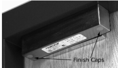
Figure 18. Installing the Tamper Finishing Caps
