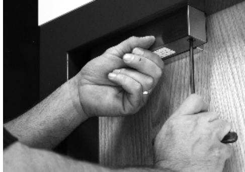
Figure 17. Installing the Magnalock
