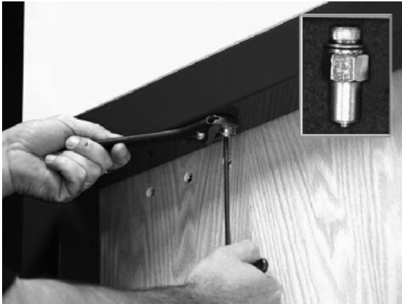
Figure 9. Installing the Blind Nuts
