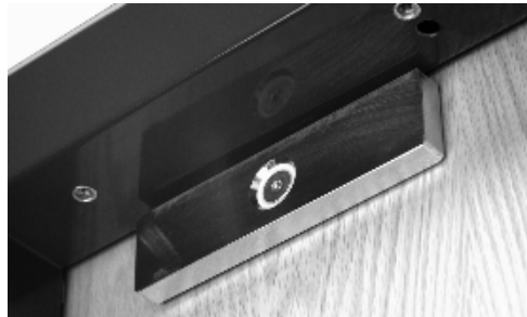
Figure 16. Installing the Strike Plate
