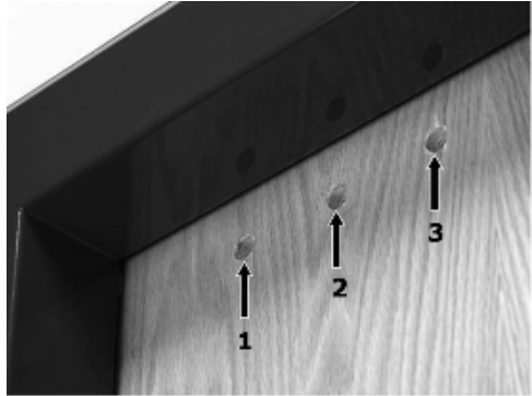
Figure 6. Installation Drill Holes
