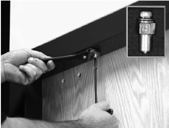
Figure 9. Installing the Blind Nuts
